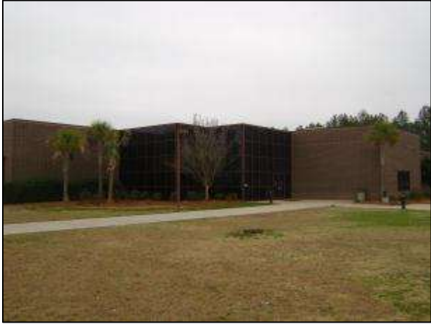
View of Library. 25 Ton RTU located on the left wing, and 20 Ton RTU located on the right wing.
